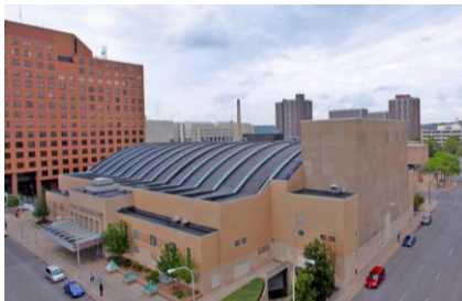
High ceilings and lack of access made re-circuiting or running control wiring impractical.
